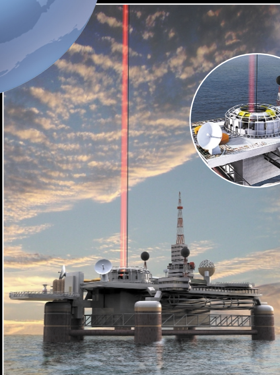
ELEVATOR AHOY: The space elevator would be anchored to Earth by a floating platform, located on the equator several hundred kilometers west of the Galápagos Islands. The platform would also house lasers used to power the elevator cars. Its mobility would allow the elevator cable to be moved out of the way of orbiting objects.
